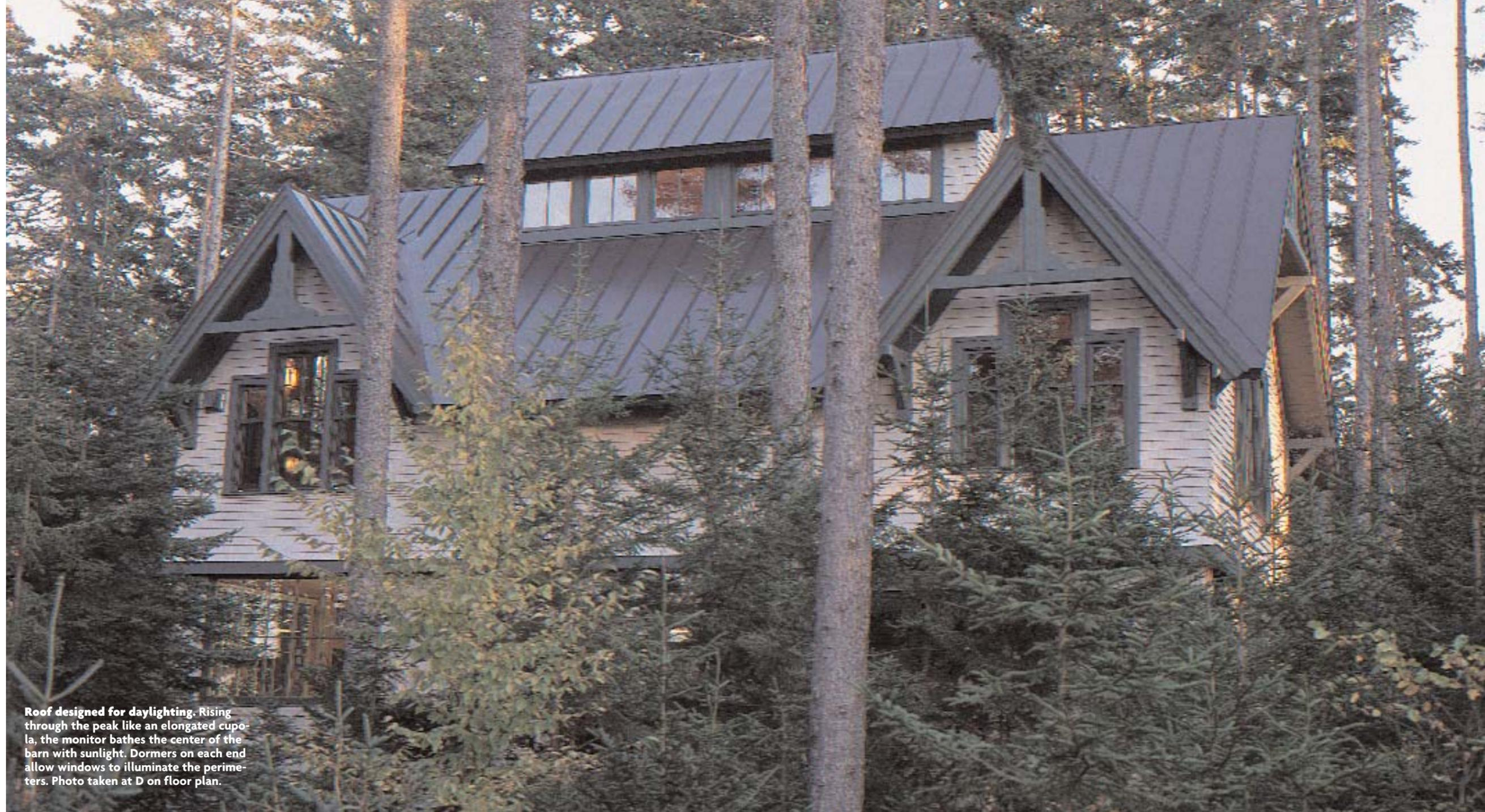
**Roof designed for daylighting.** Rising through the peak like an elongated cupola, the monitor bathes the center of the barn with sunlight. Dormers on each end allow windows to illuminate the perimeters. Photo taken at D on floor plan.
