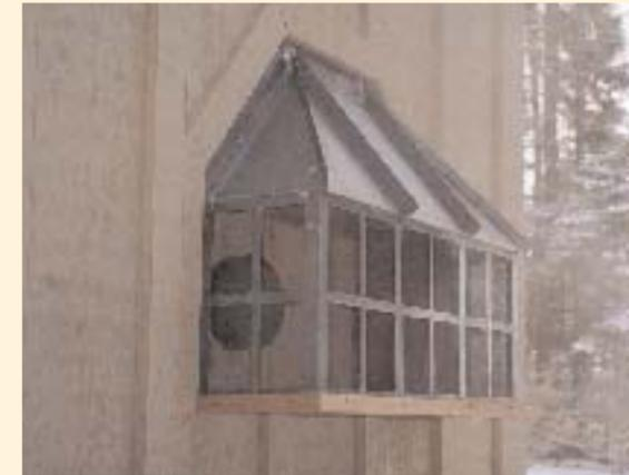
**Creative deception.** Designed to resemble Craftsman-style light fixtures, a custom-built cover conceals the heating system's intake and exhaust pipes. Photo taken at F on floor plan.
